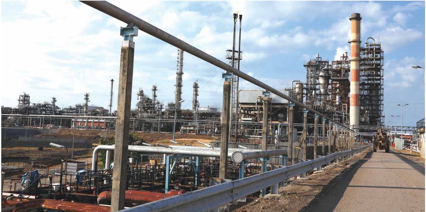
HRC's refinery in Port Dickson.
