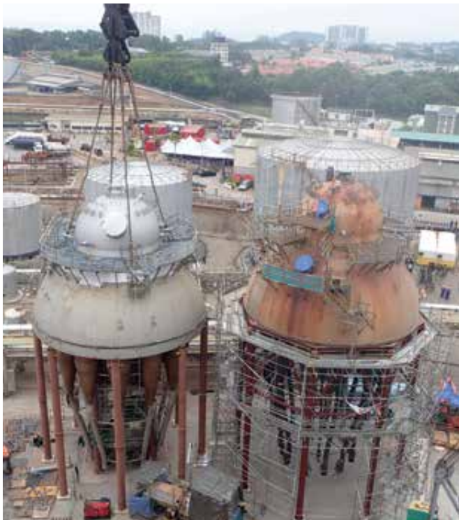
Project ATLAS II – Replacement of LRCC regenerator top dome.
