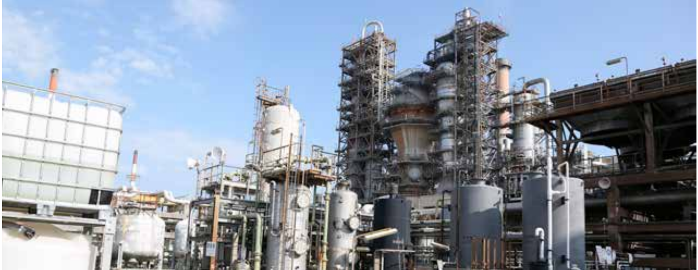
MTA 2018 was completed successfully with a good safety performance.
